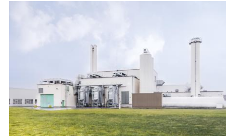
District heating plant with ICE
